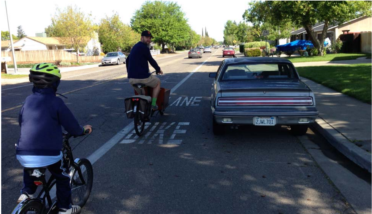
Figure 10: A typical 13' wide shared bike / parking lane in Turlock, showing bicyclists at edge of door zone
