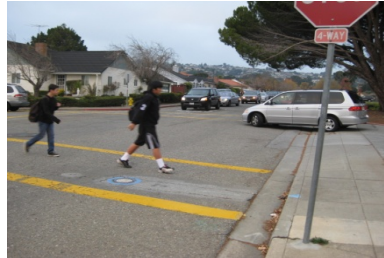
Transverse crosswalks have latitudinal lines.
