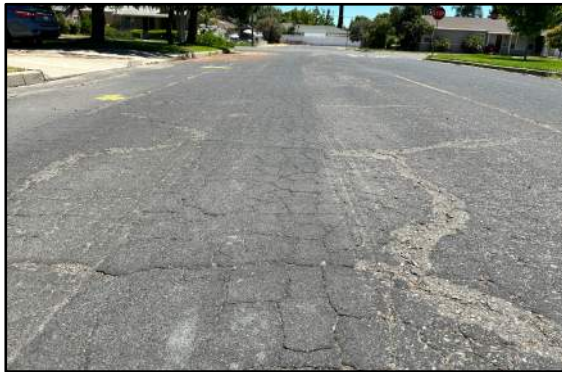
Photos 5 & 6: High severity alligator cracking propagating through delaminating slurry seal.
