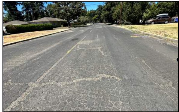
Photos 5 & 6: High severity alligator cracking propagating through delaminating slurry seal.
