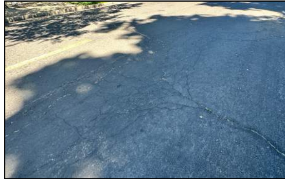
Photo 13: Low severity rutting at potential dig out.
