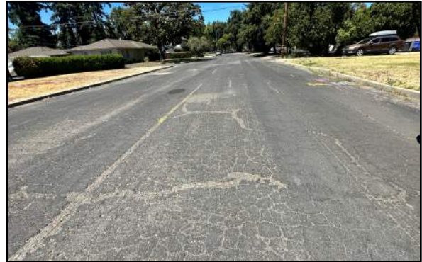
Photos 5 & 6: High severity alligator cracking propagating through delaminating slurry seal.
